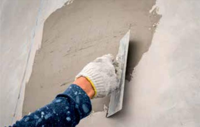
Figura 107 - Barramento final com ARGAMASSA THERMINNOV
